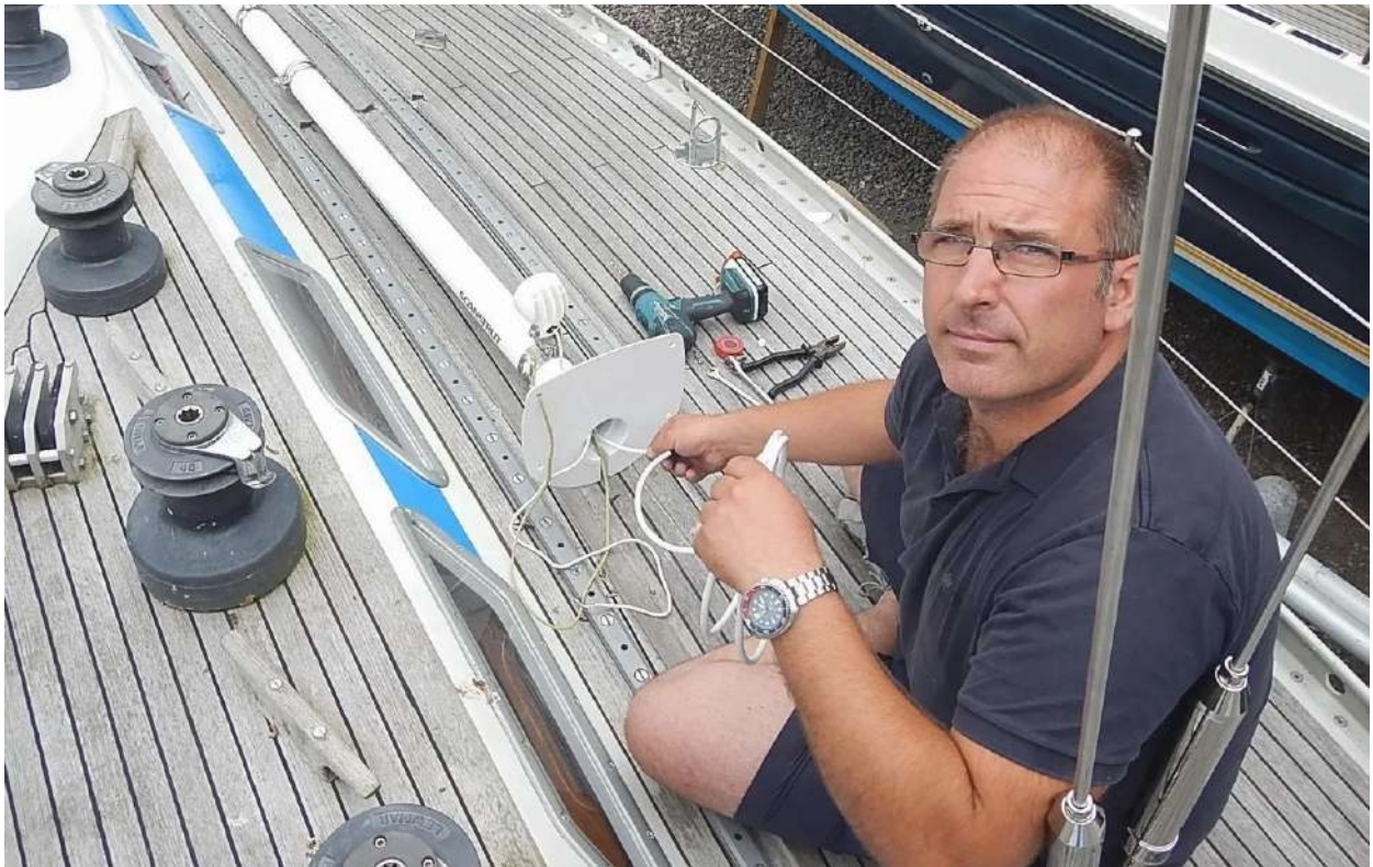
Pole assembly , pulling the radar and deck light wires through the recessed conduit
