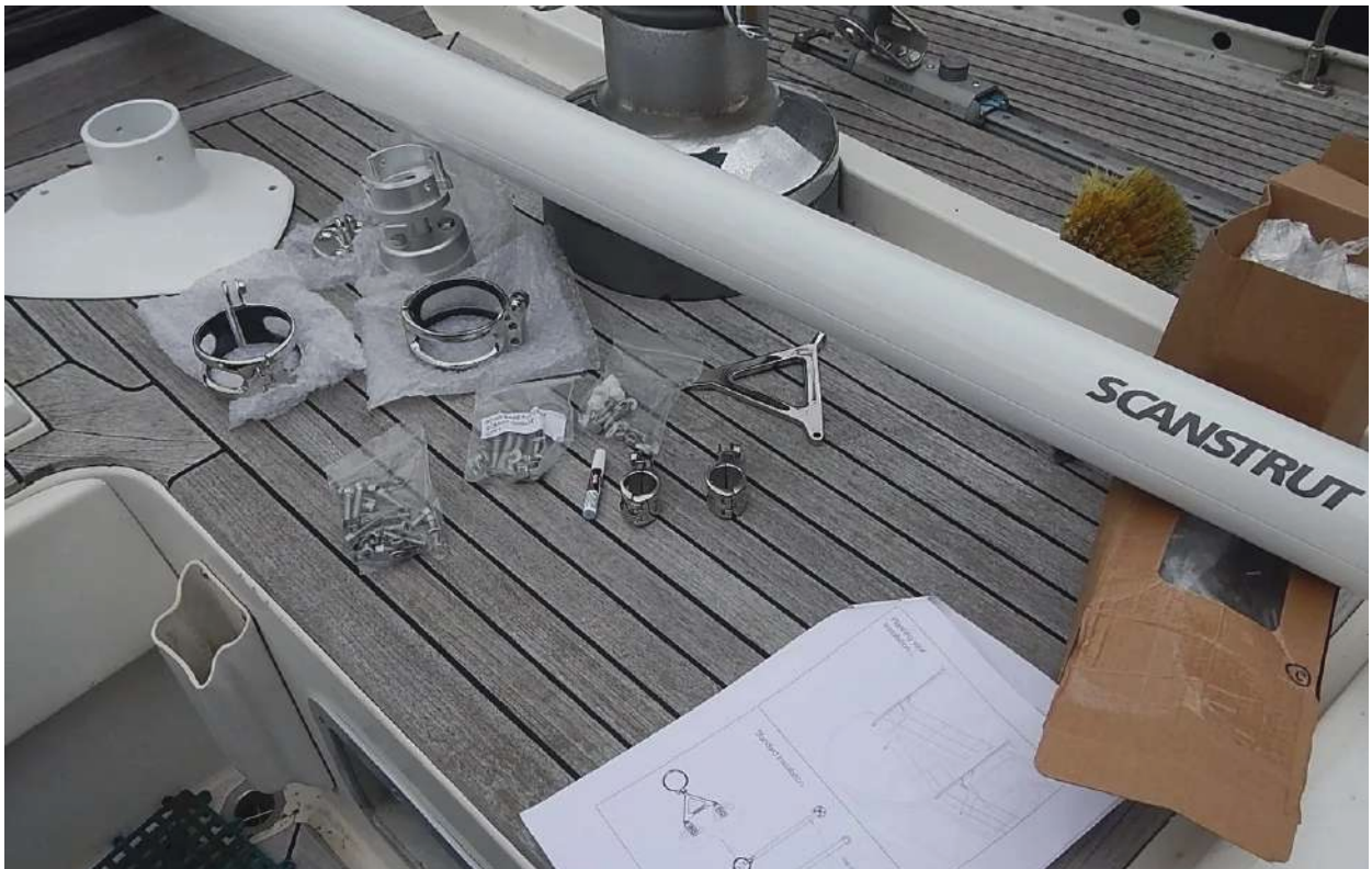
We laid out all the fittings on the deck to check we had everything we needed to complete the job.
